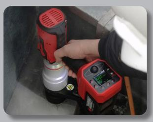
The connected steelwork must be within certain tolerances on position and straightness, but must also conform in terms of the bolting process used. The EvoTorque® Battery Tool can perform a multistage tightening sequence, where
